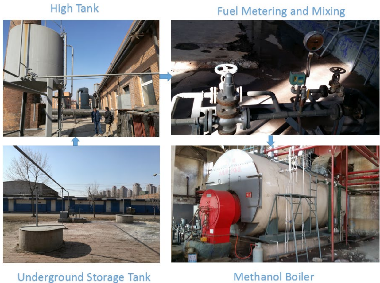
Figure 1-6 A 15 t/h Methanol Boiler for a Musical Instrument Plant in Tianjin
